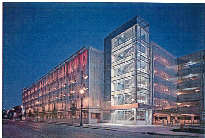
METAL SCREENS AT GARAGE, GLOWING CLUBHOUSE
