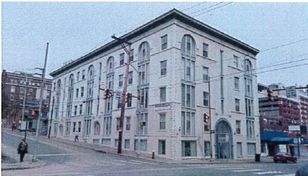
ADJACENT BUILDING - 3401 FORBES AVE
